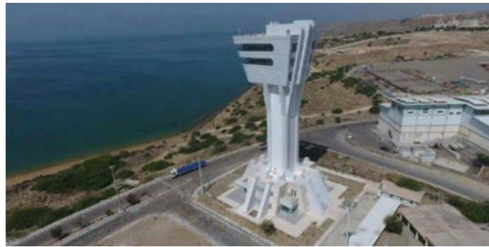
Figure 5: MRCC Chabahar, following direct impact and destruction of the operational section.
