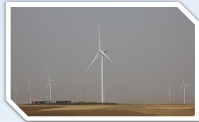
55 MW Wind farm (Takestan, Qazvin Province, Iran)
