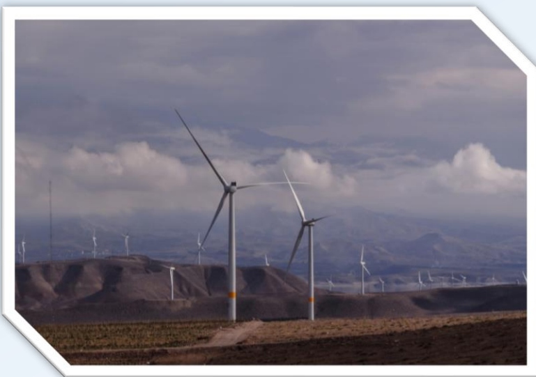
61.2 MW Wind farm (Qazvin Province, Iran)
